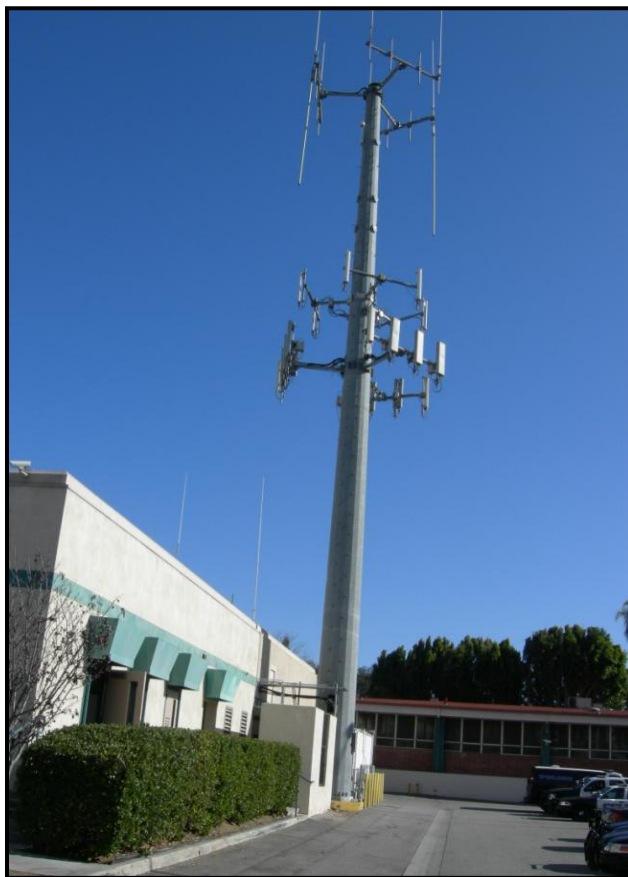
Figure 2.1-5 Typical Undisguised Monopole
