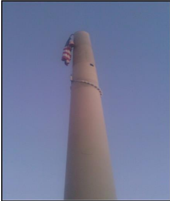
Monopole disguised as flagpole
