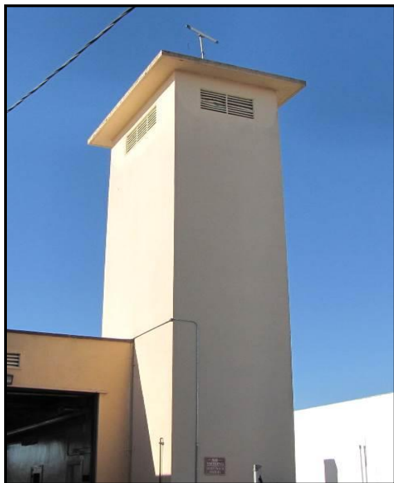
Monopole disguised as a “hose tower” at a fire station
