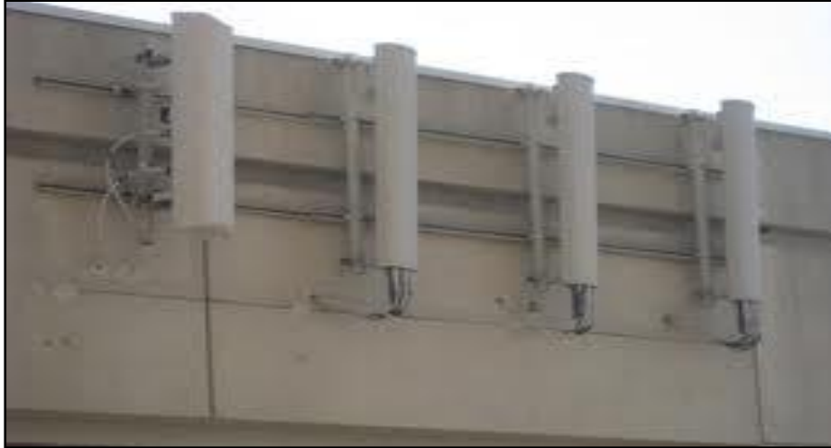
Figure 2.1-9 Example of Wall-mounted Broadband Panel Antennas
