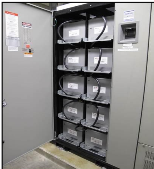
Figure 2.1-11 Batteries for Backup Power (Representative Illustration)
