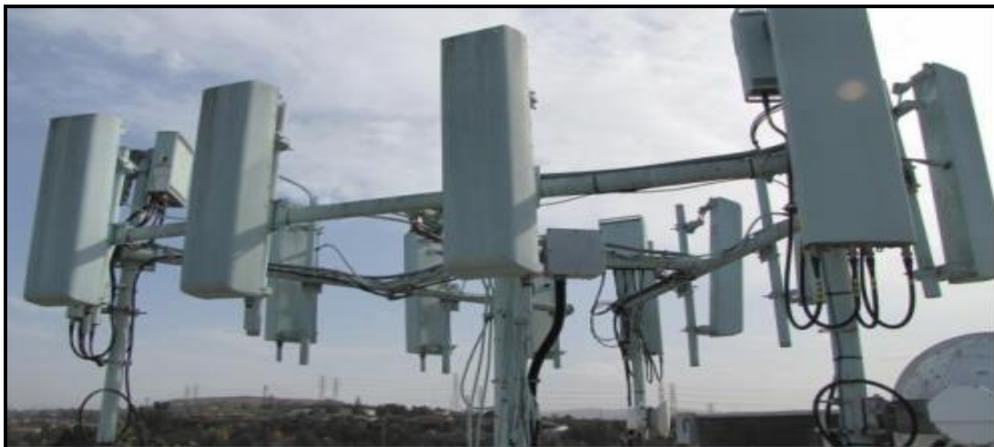
Figure 2.1-7 Example of Panel Antenna Arrays on T-Arms
