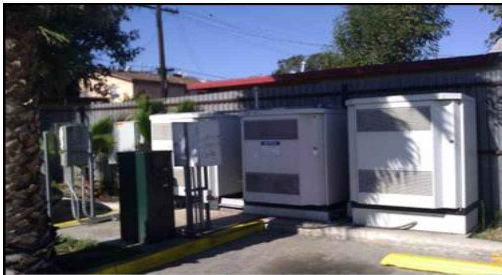
Figure 2.1-10 Typical Outdoor Communication Equipment Cabinets
