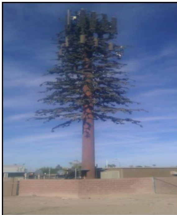
Monopole disguised as a “monopine”
