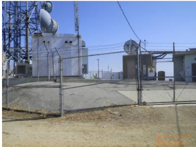
Site view looking north
