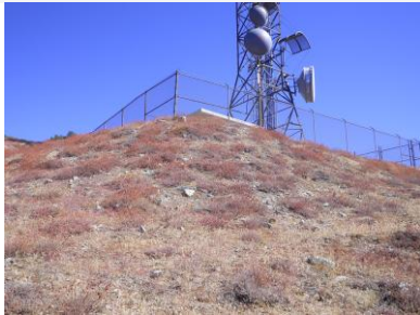
Site view looking north
