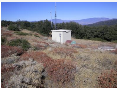
Site view looking west
