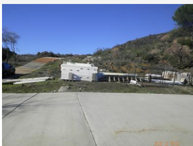
Site view looking west
