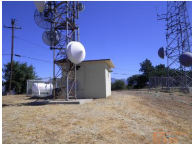
Site view looking north
