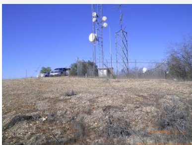
Site view looking west
