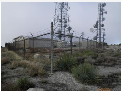
Site view looking west
