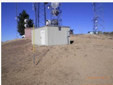
Site view looking west
