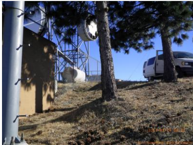
Site view looking north
