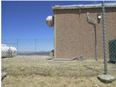
Site view looking north
