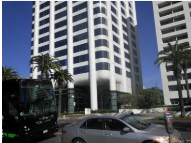
Site view looking north
