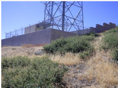
Site view looking south
