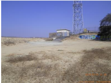
Site view looking north
