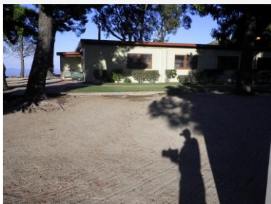
Site view looking west
