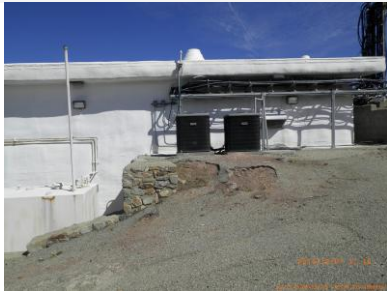
Site view looking north
