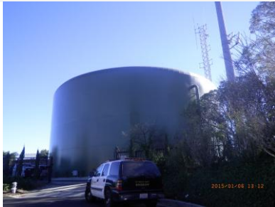
Site view looking north
