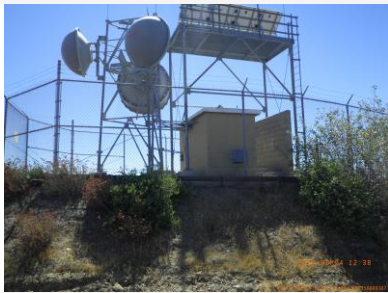
Site view looking south
