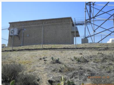
Site view looking west
