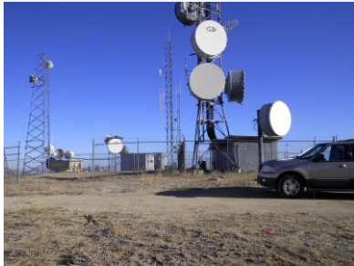
Site view looking north
