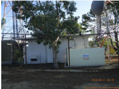
Site view looking north
