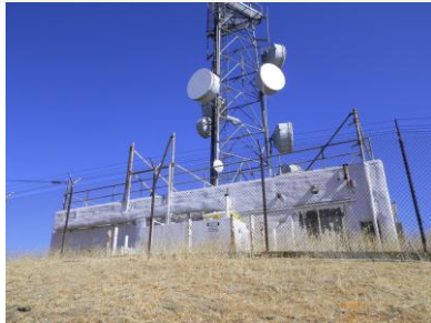
Site view looking north
