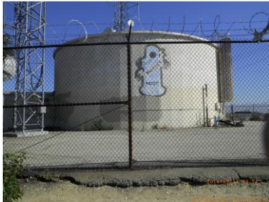
Site view looking north
