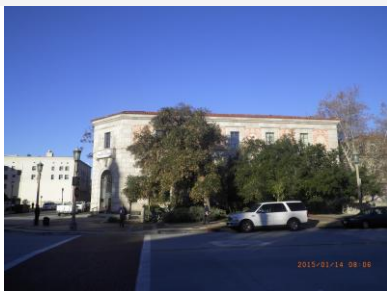
Site view looking west
