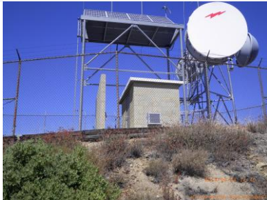
Site view looking north
