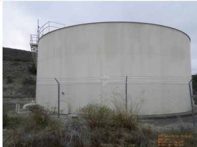
Site view looking north
