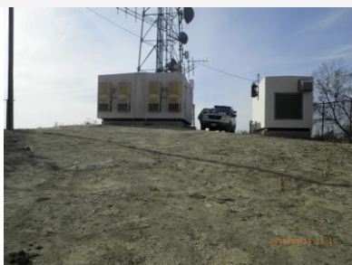
Site view looking west
