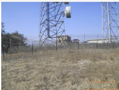
Site view looking west
