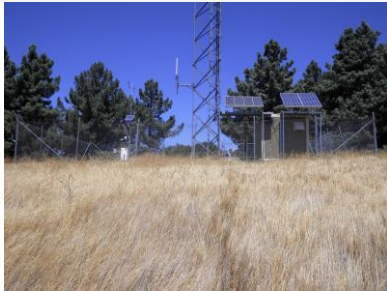
Site view looking north
