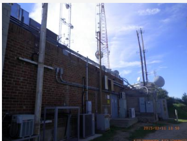
Site view looking west
