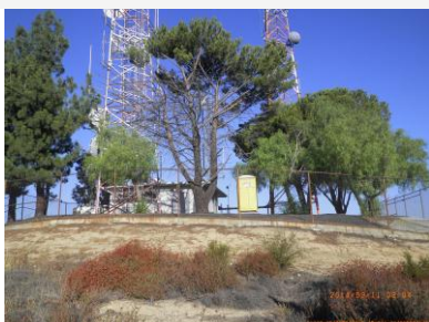
Site view looking west
