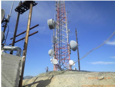
Site view looking north
