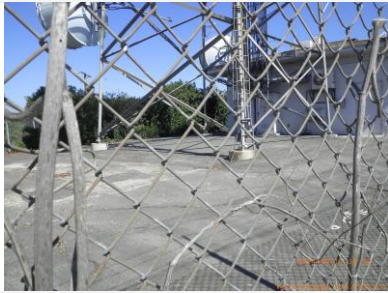
Site view looking north
