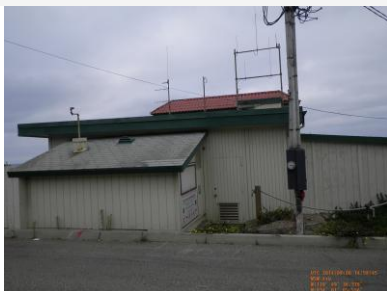
Site view looking west
