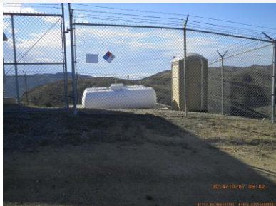
Site view looking south
