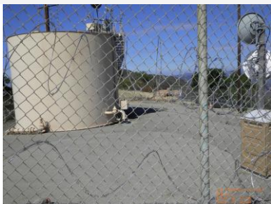
Site view looking west
