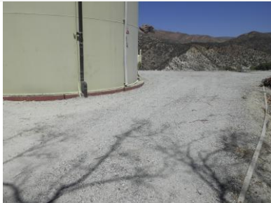
Site view looking north
