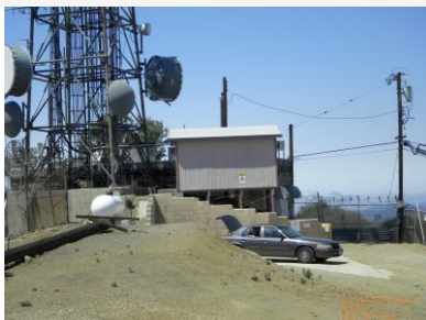
Site view looking west
