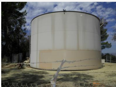
Site view looking west
