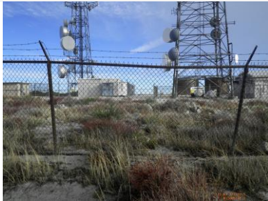
Site view looking north
