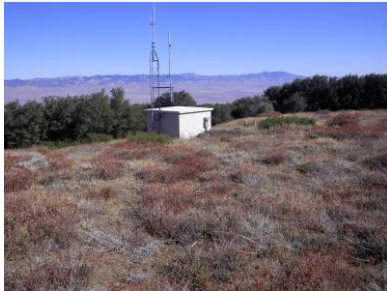
Site view looking north
