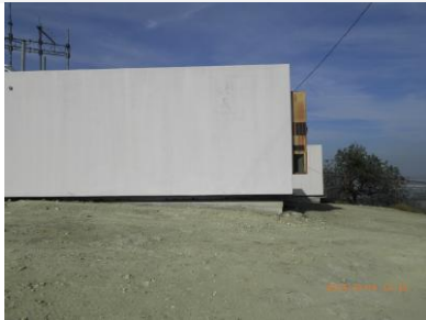
Site view looking north
