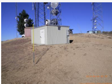
Site view looking west
