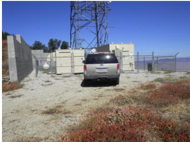
Site view looking north
