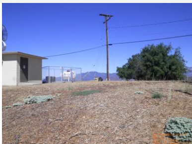
Site view looking west
