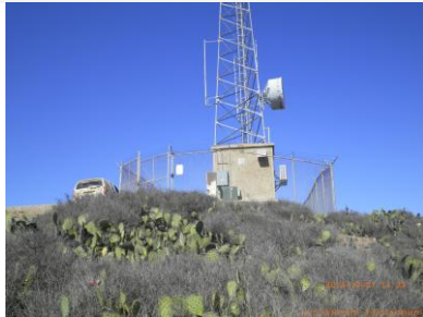
Site view looking north
