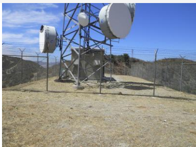
Site view looking west
