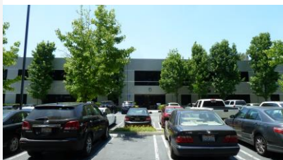
Site view looking west
