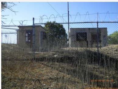
Site view looking south
