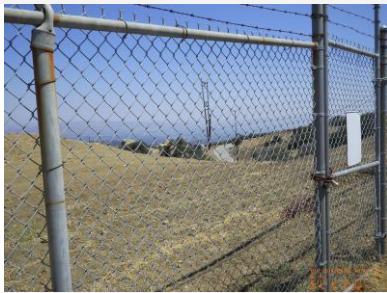
Site view looking south
