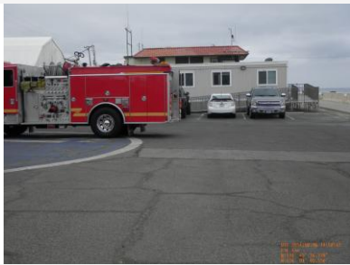
Site view looking south
