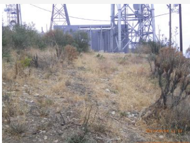
Site view looking west
