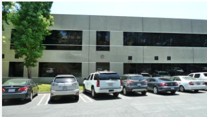
Site view looking south
