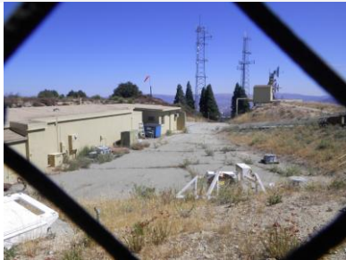
Site view looking north
