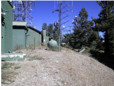
Site view looking north
