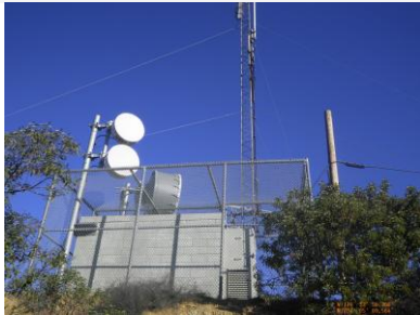
Site view looking north
