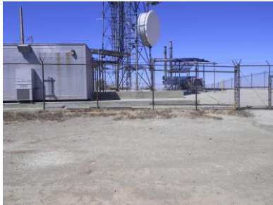
Site view looking north
