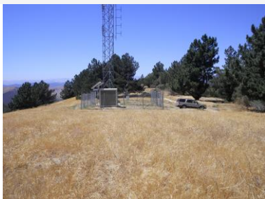
Site view looking west
