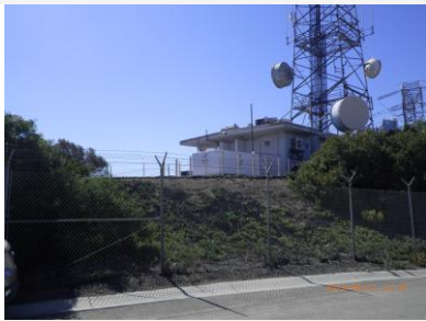
Site view looking south
