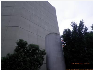
Site view looking west
