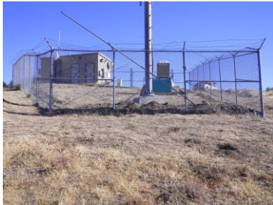
Site view looking north
