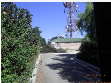
Site view looking west
