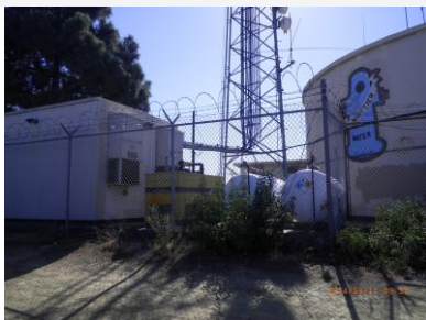
Site view looking west
