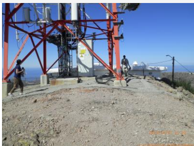
Site view looking west
