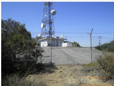
Site view looking west
