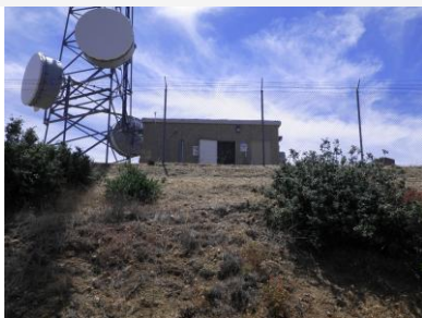
Site view looking south
