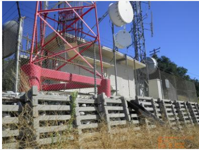
Site view looking north
