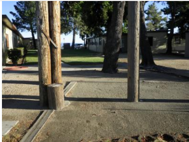
Site view looking north
