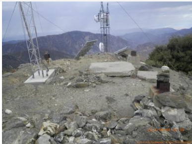
Site view looking west
