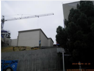
Site view looking north
