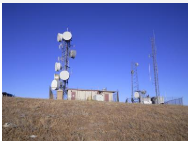
Site view looking west
