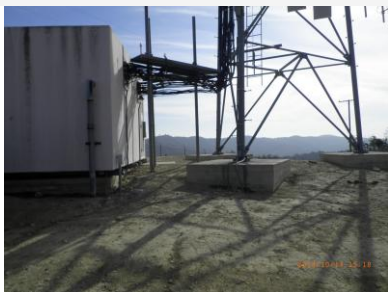
Site view looking south
