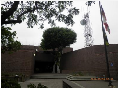
Site view looking north
