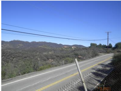
Site view looking north
