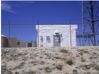
Site view looking north
