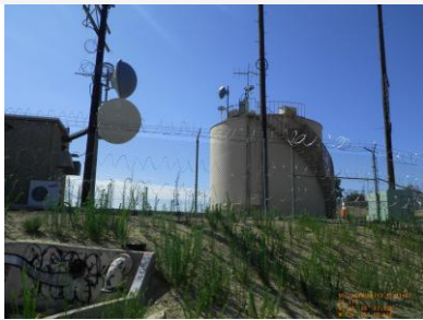
Site view looking south
