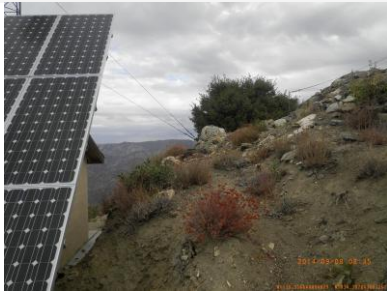
Site view looking north
