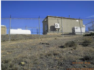
Site view looking north
