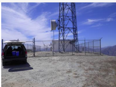
Site view looking west
