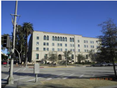
Site view looking north
