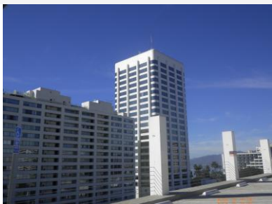
Site view looking west
