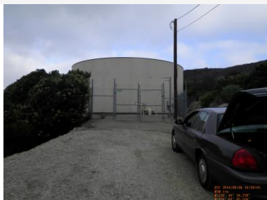
Site view looking west
