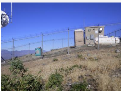
Site view looking west
