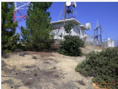
Site view looking west
