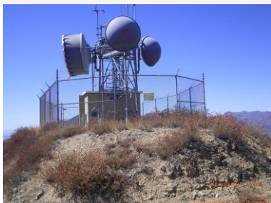
Site view looking west
