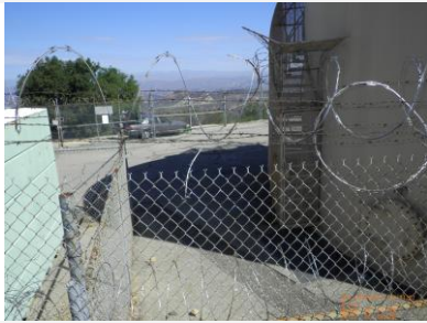
Site view looking north
