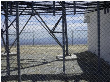
Site view looking south
