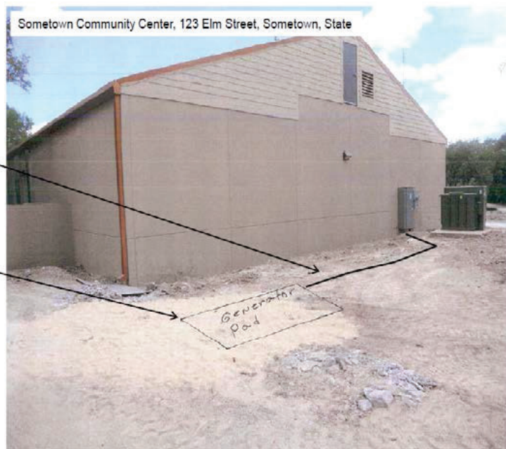
Figure 4. Ground-level photograph showing proposed ground disturbance area.
