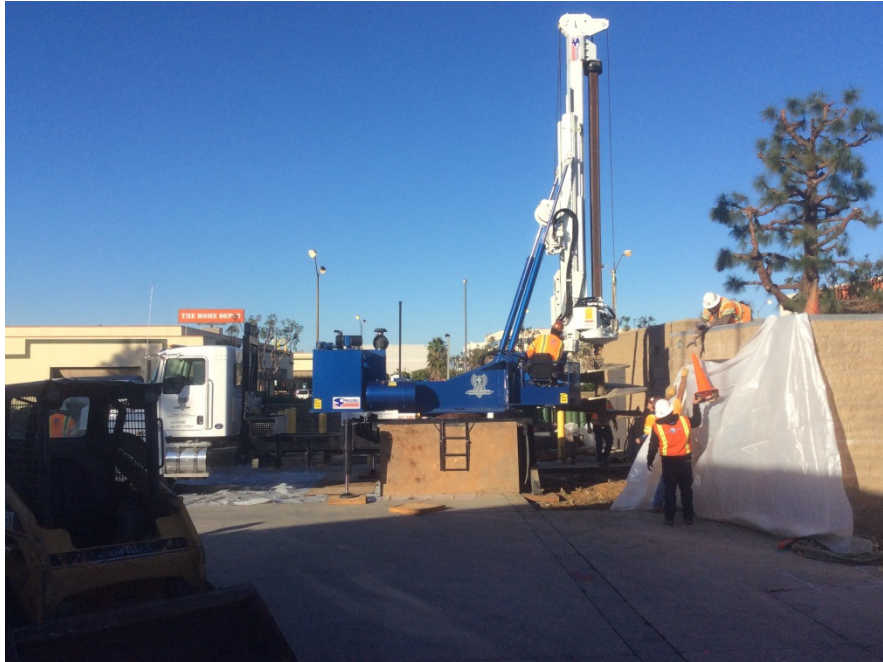
Figure 7: Example of Auger Equipment and Activity that may be used at PSBN Sites LDWP243 and ONK
